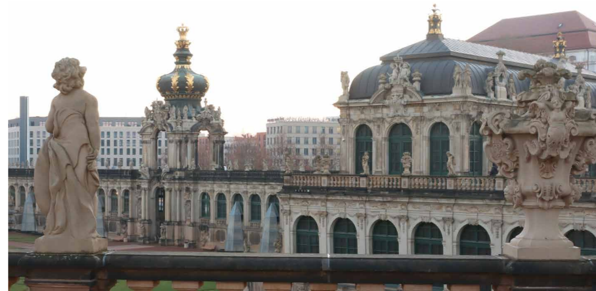
Fig. 6a, b Facade proportions influenced by patinated architecture, below: restored attic and balustrade sculptures. [Zwingerbauhütte, 1999 / 2025]
