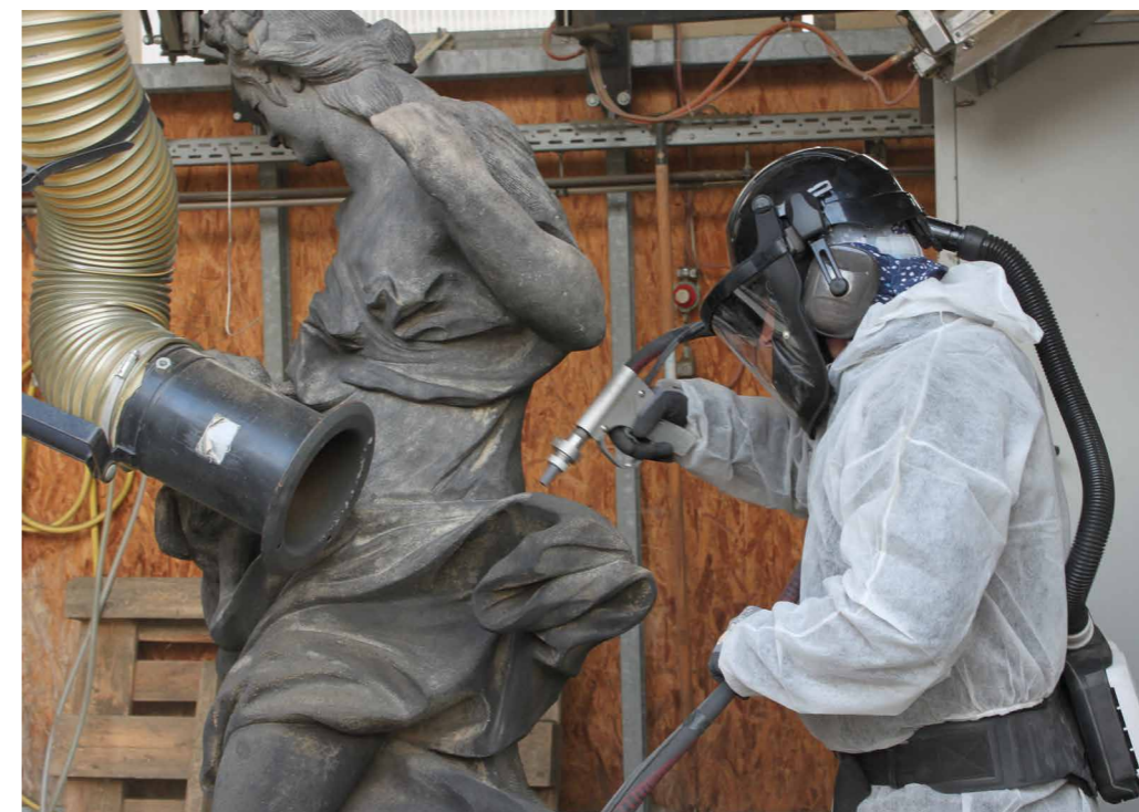
Fig. 4 Low pressure glass powder blasting in order to carefully thin compacted patina areas. [Zwingerbauhütte, 2016]
