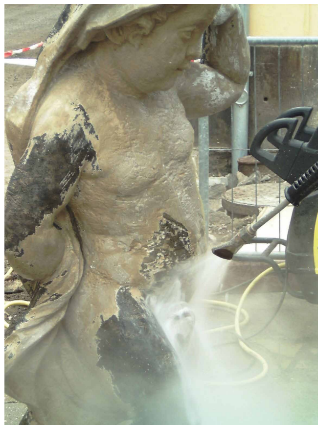
Fig. 5 Reversible silicone resin paint layer, removed in steam jet method before regularly renewal. [Zwingerbauhütte, 2005]
